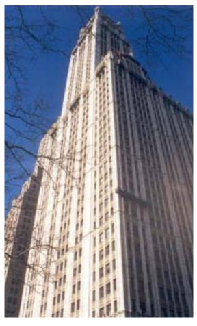
cotta cladding and ornament with new cast concrete and GFRC panels to match as closely as possible the original building appearance. Restoration has included stabilization pinning of original terra cotta cladding, in place wherever possible, re-setting of original terra cotta stones, Continued on following page
