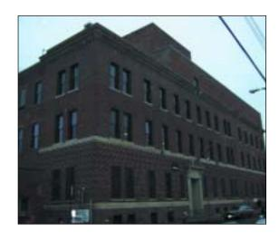
The FMD Team was responsible for replacement of cracked and displaced face brick, partial replacement of displaced parapet walls, patching and replacement of deteriorated limestone ornamentation, pointing of deteriorated mortar, the replacement of corroded structural steel, and repair of deteriorated structural concrete at the sidewalk vault structure.
