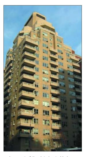
replacement of the deteriorated balcony railing system, pointing of deteriorated mortar, and the repair of corroded structural steel.
