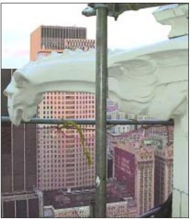
re-pointing of mortar joints, patching of original terra cotta glaze material and repair and replacement of corroded structural steel as required, in addition to the repair and replacement of copper and bituminous roofing wherever necessary. FMD also designed unique flashing and anchorage details and restored missing ornamentation and color schemes.
